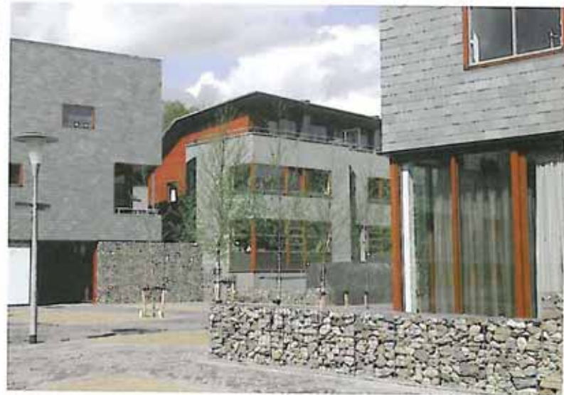
Schanskorven in de gevels en langs de randen van de kamers. Gabions in the walls and along the edges of the 'rooms'.
