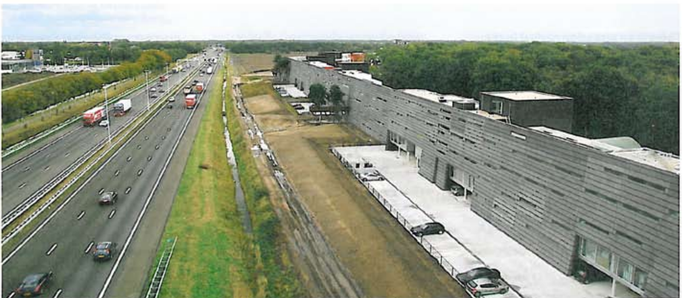
The screen barrier along the A58 motorway, designed by Bureau Lubbers and Crepain-Binst Architecture.
